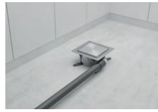
2. The adjustable legs (optional additional payment) should be glued in the places shown. Connect the point drain to the drainage system and set thie height using the adjustable legs so that the upper edge of the frame is approximately 1mm below the finished surface level of the shower. We recommend that you do not remove the protective foil from the grating until the installation is complete.
