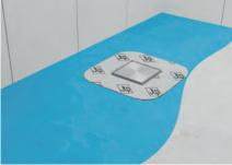
5. Unfold the membrane and slightly press it to the wet foil to ensure close adherence.
