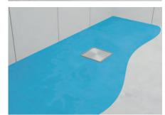
4. Cover the flange and the surrounding area with an insulating foil in a liquid form.
