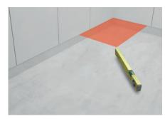
1. Set the level of the finished shower floor surface and mark it on the wall in the area where the channel will be fitted (allow for the slope of the shower surface).
